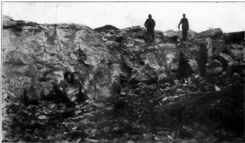
Beginning the New Quarry Drilling with Jack Hammers
